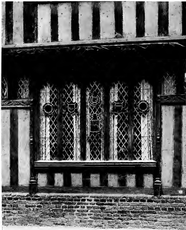
OLD OAK HOUSE, DETAIL OF WINDOW Only the small windows at either side open
